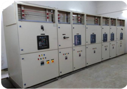
ACB Panel for Power distribution and Control up to 6000A
